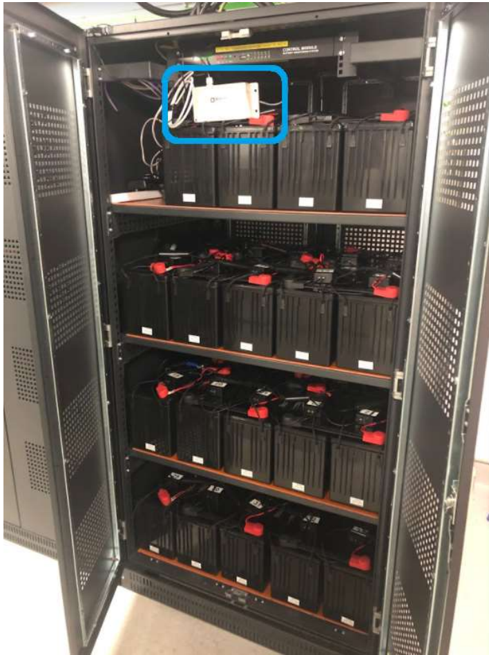
LoRaWAN Battery Monitoring System in Hong Kong-Zhuhai-Macao Bridge
