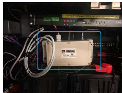
LoRaWAN Battery Monitoring System in Hong Kong-Zhuhai-Macao Bridge
